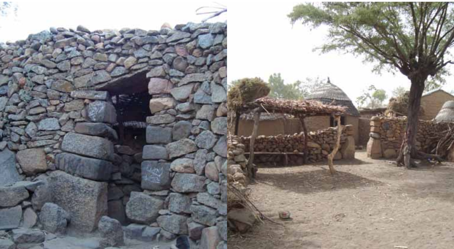
Figure 4: Left: a stone lintel over the entrance door of the residence of a Sakun leader. Right: the entrance of a typical Sakun residence with no lintel. © I. Odiava
