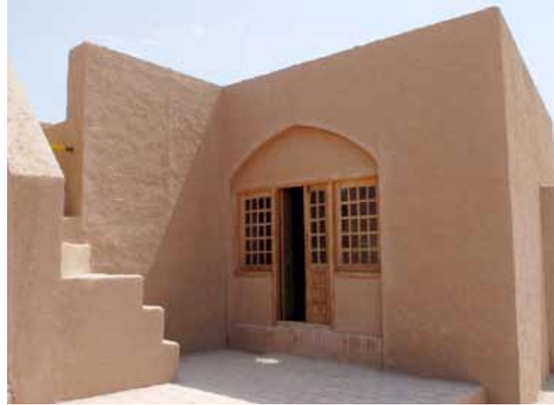
Figure 4: The Payambar Mosque after restoration.
