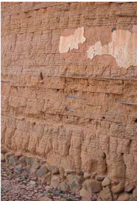
Figure 6: Features of tulou construction: a stone basement wall showing the bamboo wall bones. Source: http://amuseum.cdstm.cn/AMuseum/hakla/image/jianzhuljianzhu_082_1.jpg
