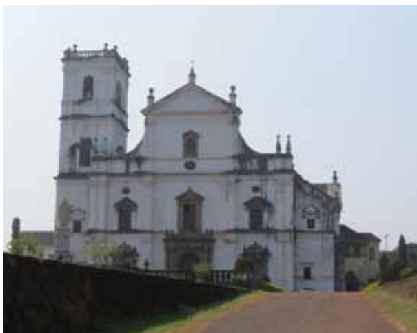
Figure 5: Front façade of Se Cathedral. Of the two towers that originally flanked the façade, the tower on the right collapsed after it was struck by lightning in 1776. © T. Sharma
