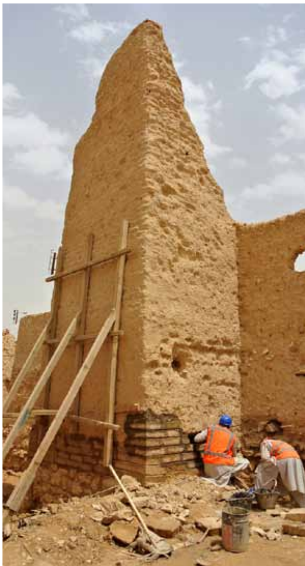
Figure 9: Pilot project: restoration works, consolidation and restoration of the wall base. © M. Bendakir
