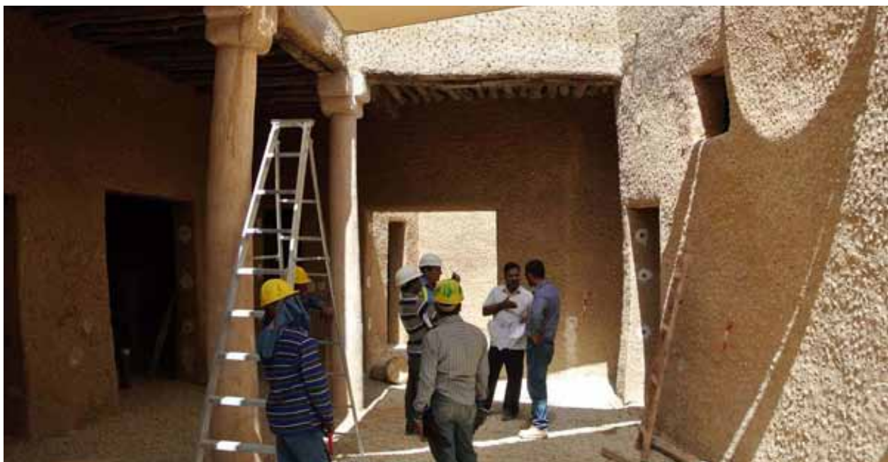
Figure 12: Pilot project: restoration works, Pilot house, courtyard canopy installation. © M. Bendakir
