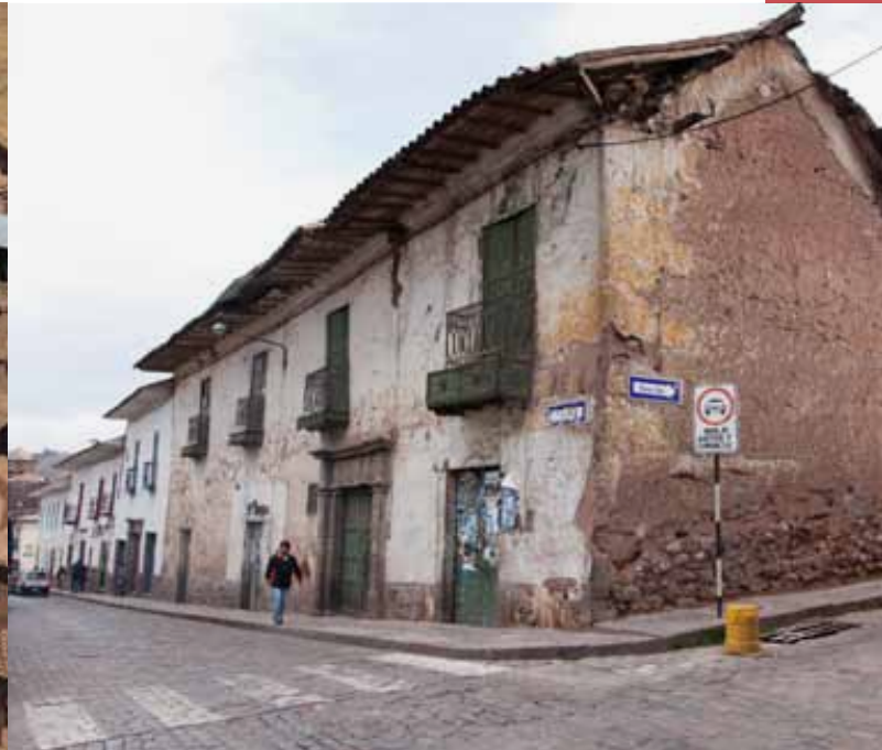
Figure 5: Facade of Casa Arones, a residential 17th-century two-story adobe and wood truss roof building in the historic center of Cusco, Peru. © Scott Warren, The J. Paul Getty Trust, 2011
