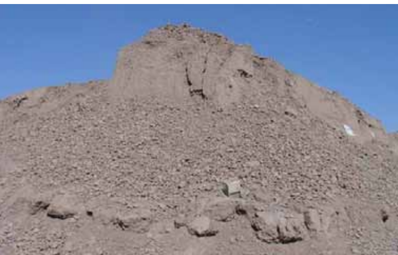
Figure 11: Ruins of Tower no. 1 immediately after the earthquake.
