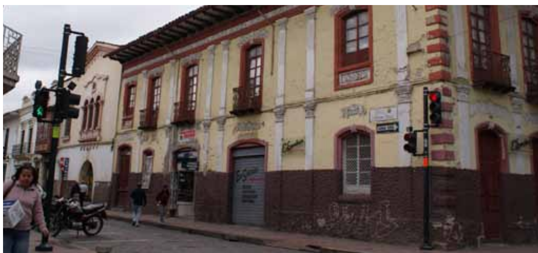
Figure 8: A historic residence on a downtown corner made of adobe and wattle and daub. © María de Lourdes Abad
