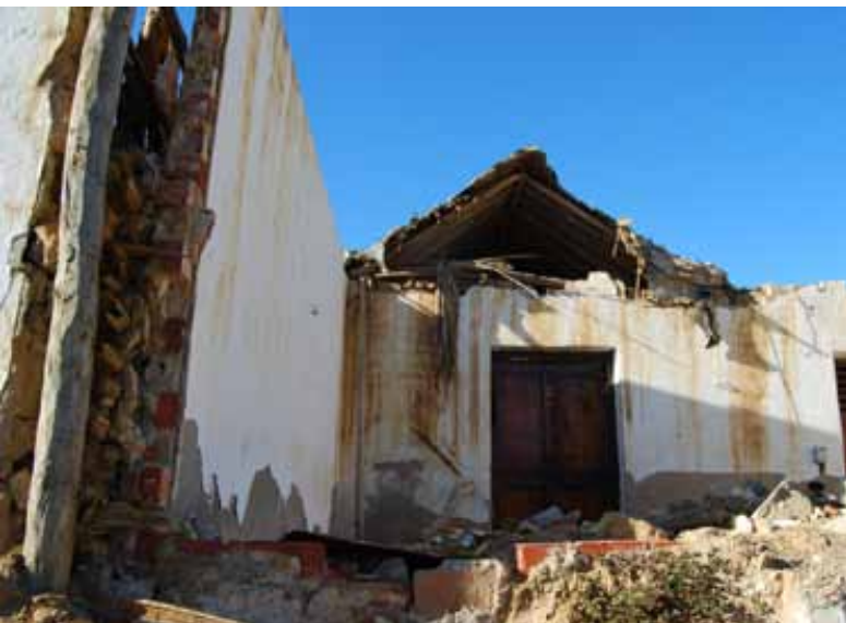
Figure 8: Use of cement-based plaster can lead to the collapse of wattle and daub walls, La Vela. © L. Guerrero
