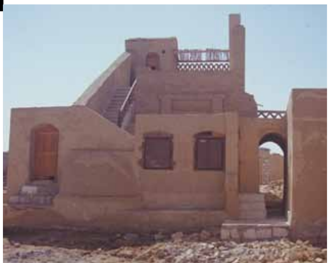
Figure 6: Eco-lodge prototype 'G' for Mr AbdAllah Schleifer, Tunness, Fayoum oasis. Egypt. 1992-93. The northern façade shows the entry tunneled corridor that acts as a suction wind shaft for all openings on it. This is in reflection as a little village scape within the small edifice calibrated in the fashion of the covered narrow streets of 'les Mzabes' of north Africa or the traditional oasis of the Egyptian deserts. © AHMAD HAMID ARCHITECTS
