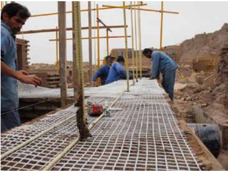
Figure 7: Using fiberglass mesh to strengthen pillars and walls.
