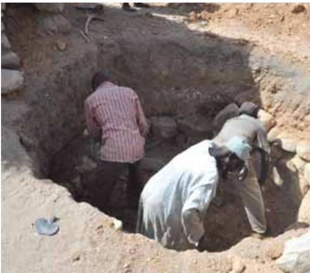
Figure 6: Construction of a sub-basement bullpen. © Michael Thomas
