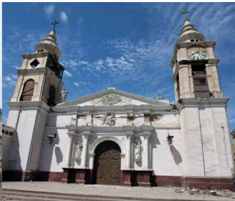
Figure 3: Facade of the 18th-century Cathedral of Ica in Peru, made of adobe and quincha vaults and domes. © Scott Warren, The J. Paul Getty Trust, 2011
