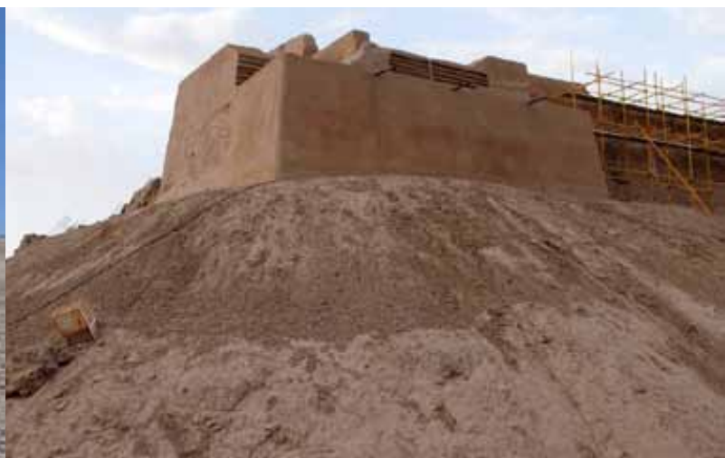
Figure 12: Tower no. 1 after restoration.
