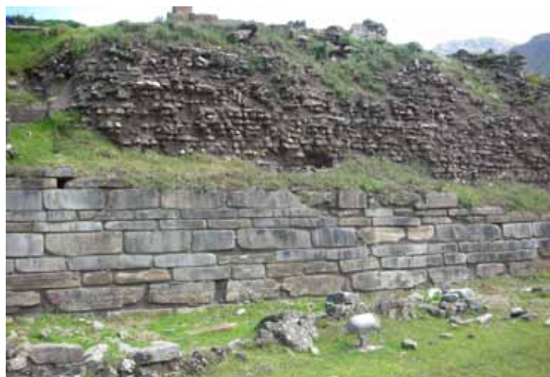
Figure 2: Chavín's solid truncated pyramids have a resistant core which has proved durable through earthquakes and other disasters, while the facades have suffered notably. © J. Vargas-Neumann
