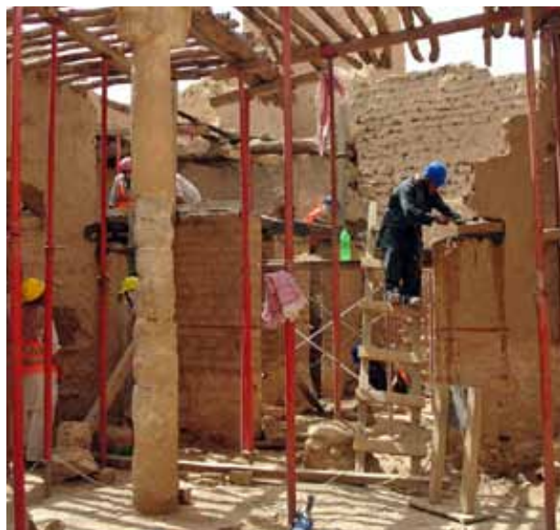
Figure 10: Pilot project: restoration works, columns restoration. © M. Bendakir
