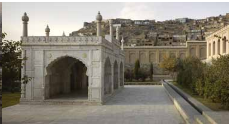
Figure 3: Baghe Babur, Kabul Mosque and perimeter wall after restoration. © Christian Richters/Aga Khan Trust for Culture
