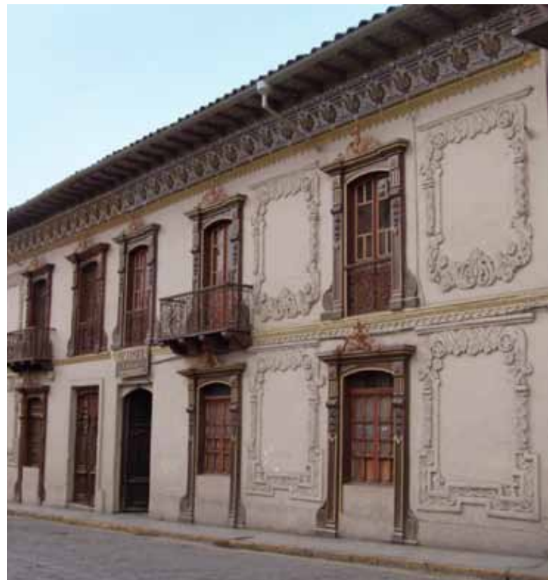
Figure 3: 'Embroidered' building, made of adobe and emphasizing decorative elements such as moulded tin ceilings, relief modelling of mud applied to outer walls, and whitewashing. © María de Lourdes Abad
