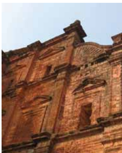
Figure 9: (L) Exposed laterite walls of the Basilica of Bom Jesus showing deterioration of the laterite blocks. (R) Water seepage from the roof affects the wall paintings inside the Church of St Francis of Assisi. © T. Sharma
