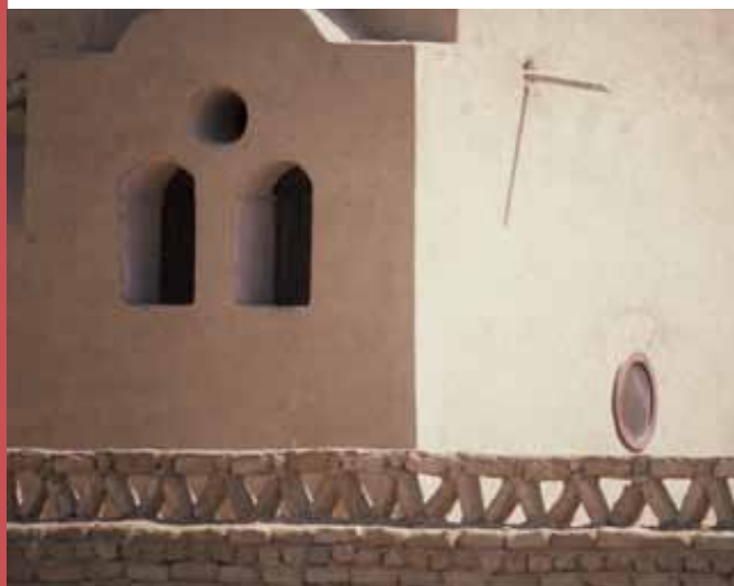
Figure 4: Eco-lodge prototype 'G' for Mr AbdAllah Schleifer, Tunness, Fayoum oasis. Egypt. 1992-93. The details of the architectural compositions are a direct and true expression of the construction process. © AHMAD HAMID ARCHITECTS
