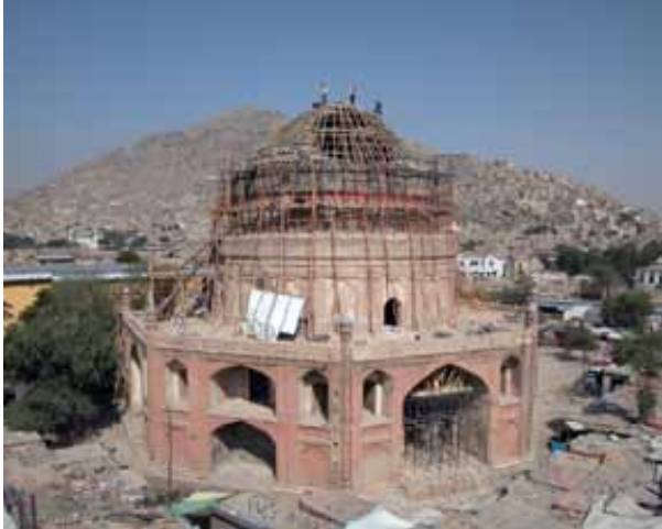
Figure 3: Timur Shah Mausoleum, Kabul, during restoration. © Aga Khan Cultural Service-Afghanistan
