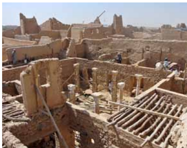
Figure 11: Pilot project: restoration works, roof reconstruction. © M. Bendakir
