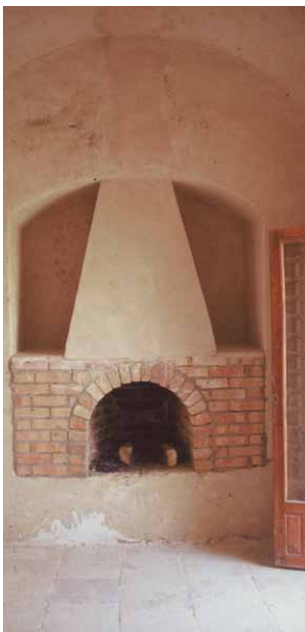
Figure 9: Eco-lodge prototype 'G' for Mr. AbdAllah Schleifer, Tunness, Fayoum oasis. Egypt. 1992-93. The interiority of the edifice shows the quality of diffused natural light, the warmth and human closeness to mud plastering. The fire place is again in respect to the structural forces implicit in its placement within the bigger structure, no décor; the lines are an outcome of an intelligent process simply. © AHMAD HAMID ARCHITECTS
