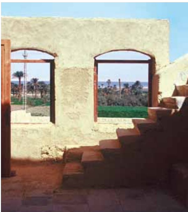
Figure 8: Eco-lodge prototype ‘G’ for Mr. AbdAllah Schleifer, Tunness, Fayoum oasis. Egypt. 1992-93. The view from the courtyard looking north to the grand lake of Quarun, is intentionally framed by two windows capturing the view bringing it in a proximate manner; and capturing as well the northern salty breeze. The stair way leading to the roof can act in an uncontrived manner as seating at the same time. © AHMAD HAMID ARCHITECTS
