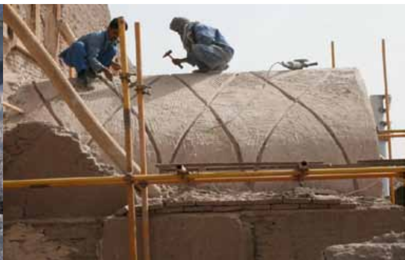
Figure 6: Strengthening an arched passage with rope made from palm fibre (SIS).
