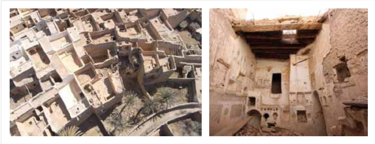
Figure 2: Abandoned houses. Left: © Grégoire Paccoud; right: © Thierry Joffroy
